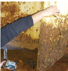
Port dock thickness measurement
